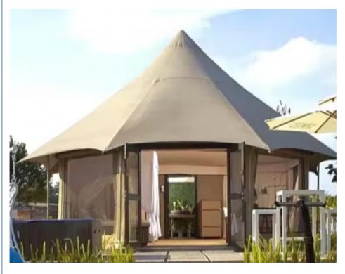
Membrane structure which called tension membrane structure ,is a new kind of building structure. It through the steel frame, steel column or wire make the membrane material produce a certain tension in order to form a certain space shape, composition can bear a certain tension stability catenary system. Membrane structure of the membrane material should be made concave and convex space curved surface to ensure its stability, so the membrane structure is called space membrane structure as well.
