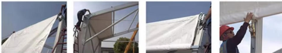
Roof Fabric Installation
