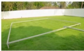
Set up the beams first
