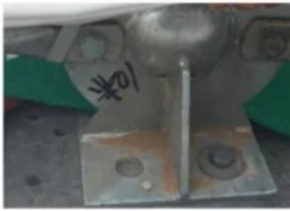
Cement floor expansion bolts be used for fixing
