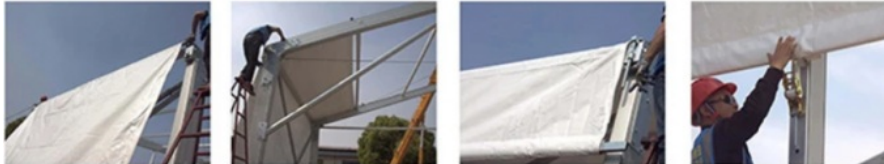
Roof Fabric Installation
