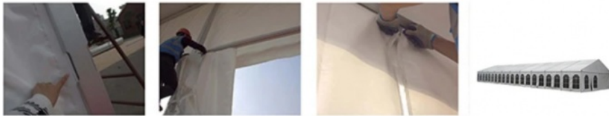
Side Wall Installation
