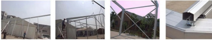
Frame Installation
