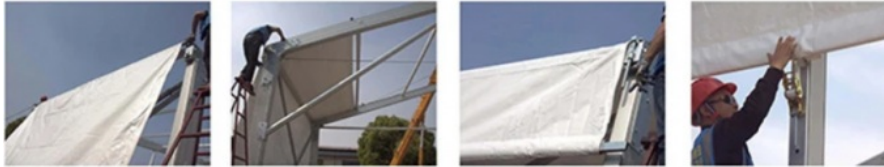
Roof Fabric Installation
