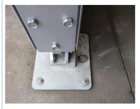
4. Bearing disk The bearing frame is secured
